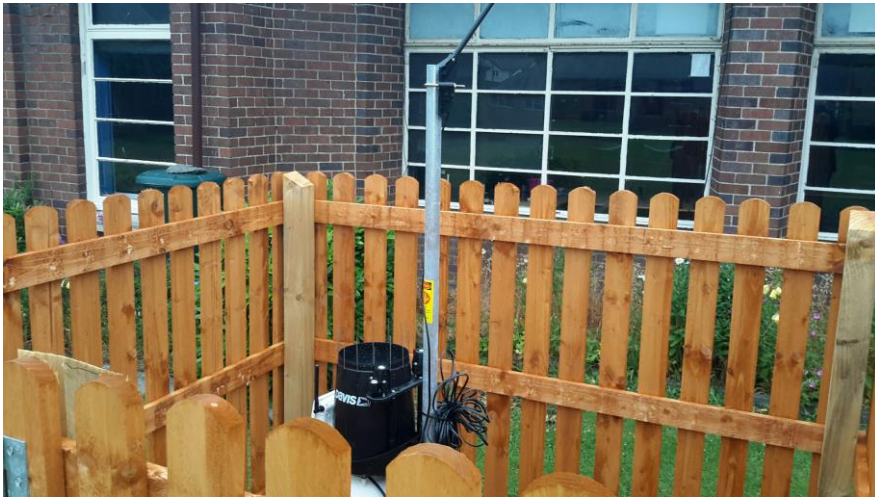
Fig. 3. Weather station node located within school grounds.
